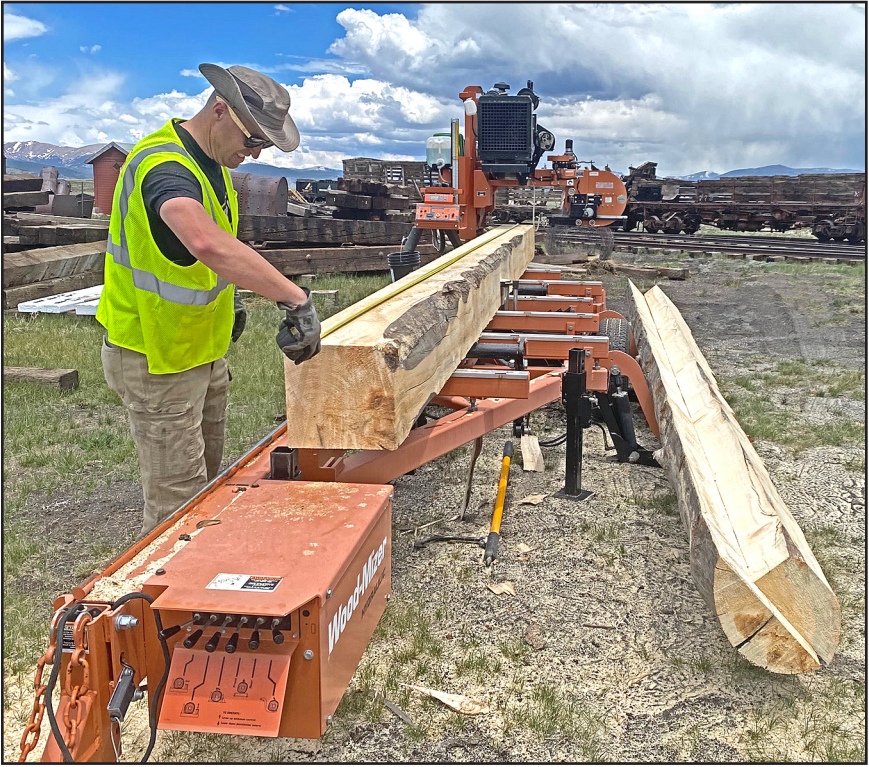
One of the main timbers for the new Como tank base being milled to size at Como. – Photo courtesy South Park Rail Society and the DSP&PHS.
