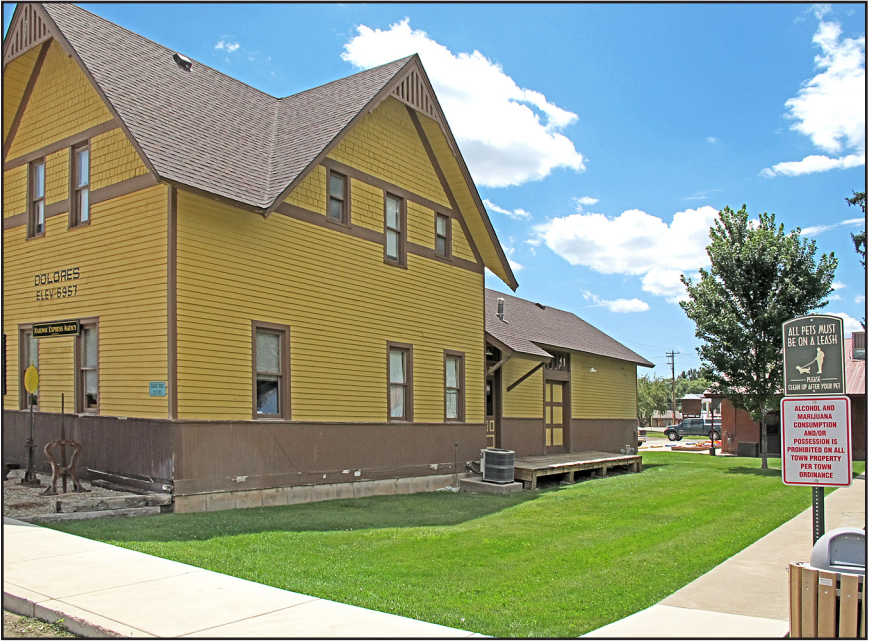
The new display track location behind the Dolores, Colorado, museum building. – Photo courtesy the Galloping Goose Historical Society.
